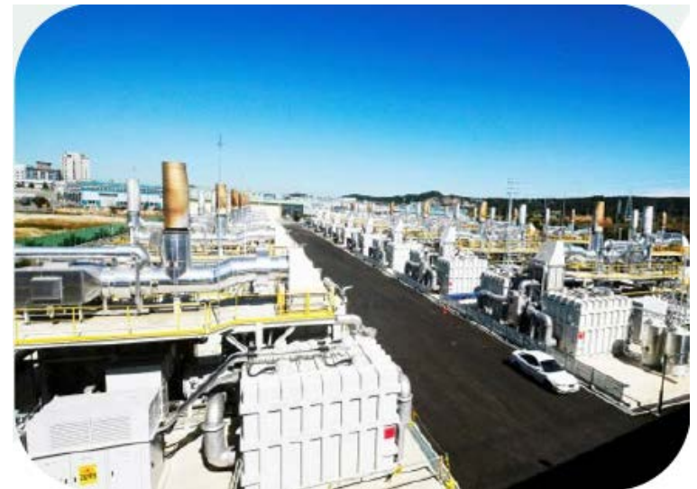
Hwaseong, South Korea 59 MW Fuel Cell System
